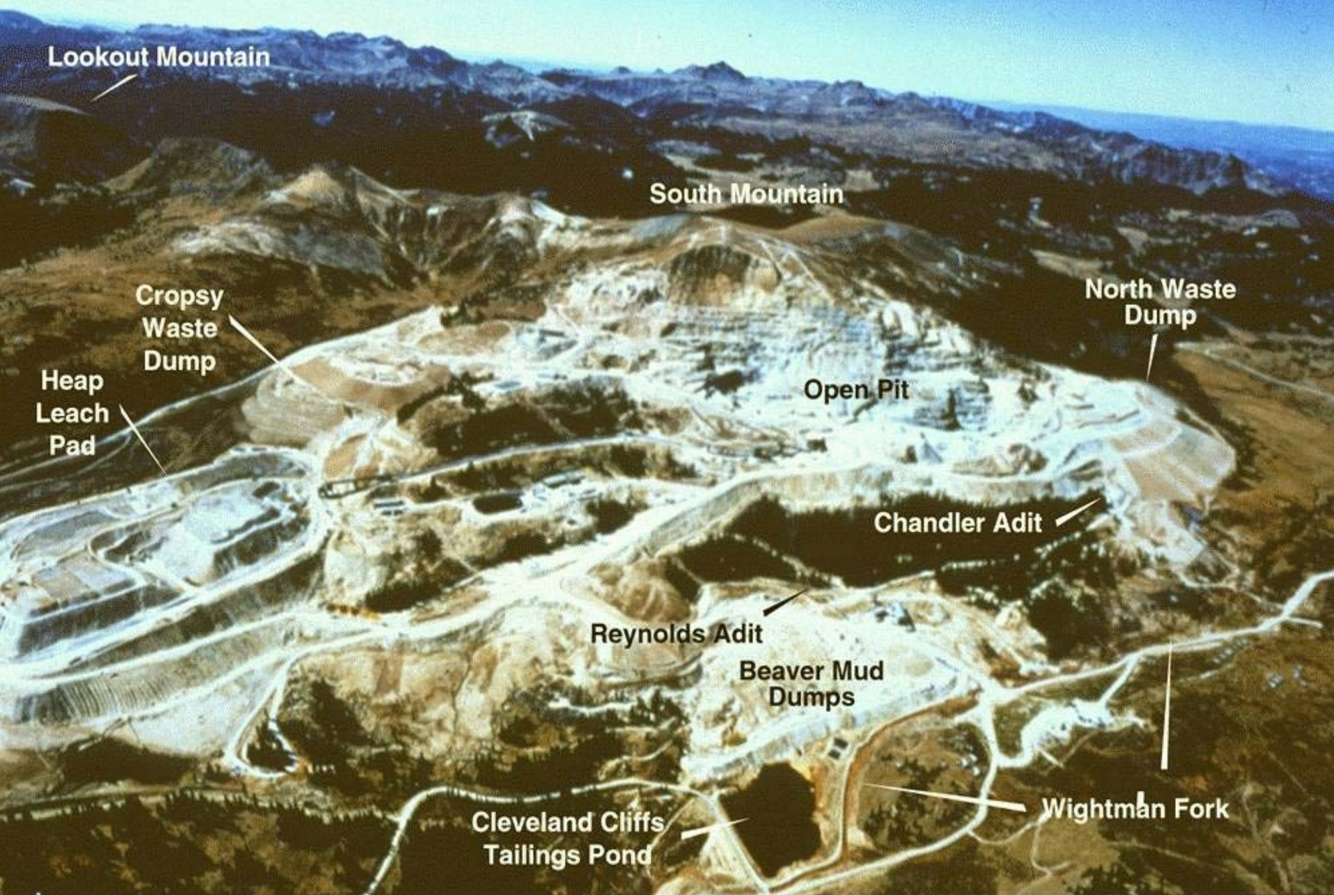
Figure 2. Oblique aerial photograph, looking south-southwest, of the Summitville Mine and vicinity. The mine is located just east of the continental divide at an elevation of 3800 meters (11,500 ft). Total yearly snowfall is approximately 7–11 meters (20–35 ft). Photo by IntraSearch, Inc.
